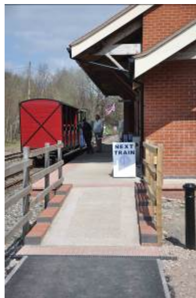
View from Point "A" in previous photo towards platform
